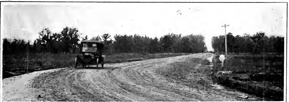
A WELL-DRAINED SURFACED ROAD IS A DISTINCT ASSET TO A COMMUNITY
